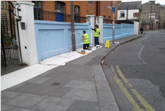
Pictured above: Work being completed on The Back Lane Hostel
